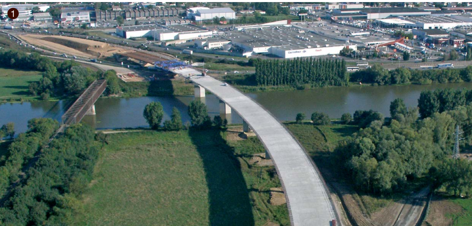
1 Construction of the viaduct over the River Maine, A11 Angers
