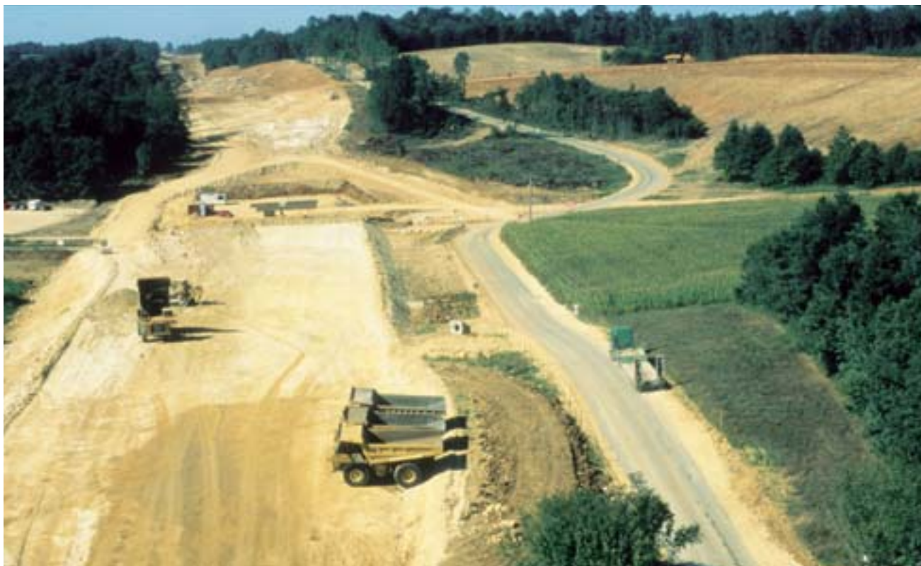
Construction of the Périgueux/Thenon section of the A89.
