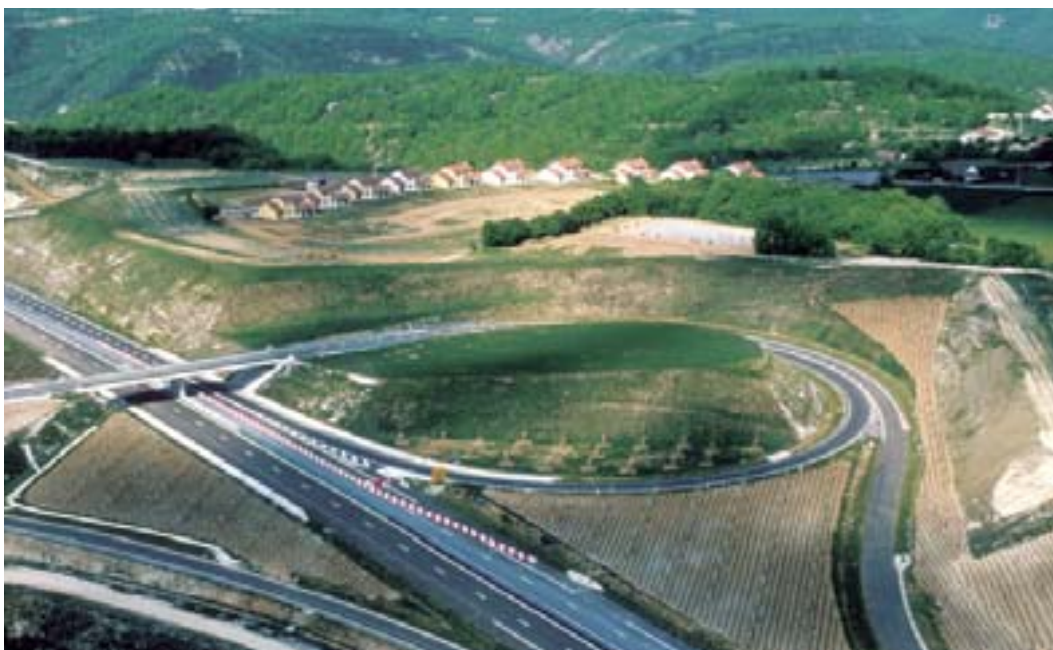
Aerial view of the A89.
