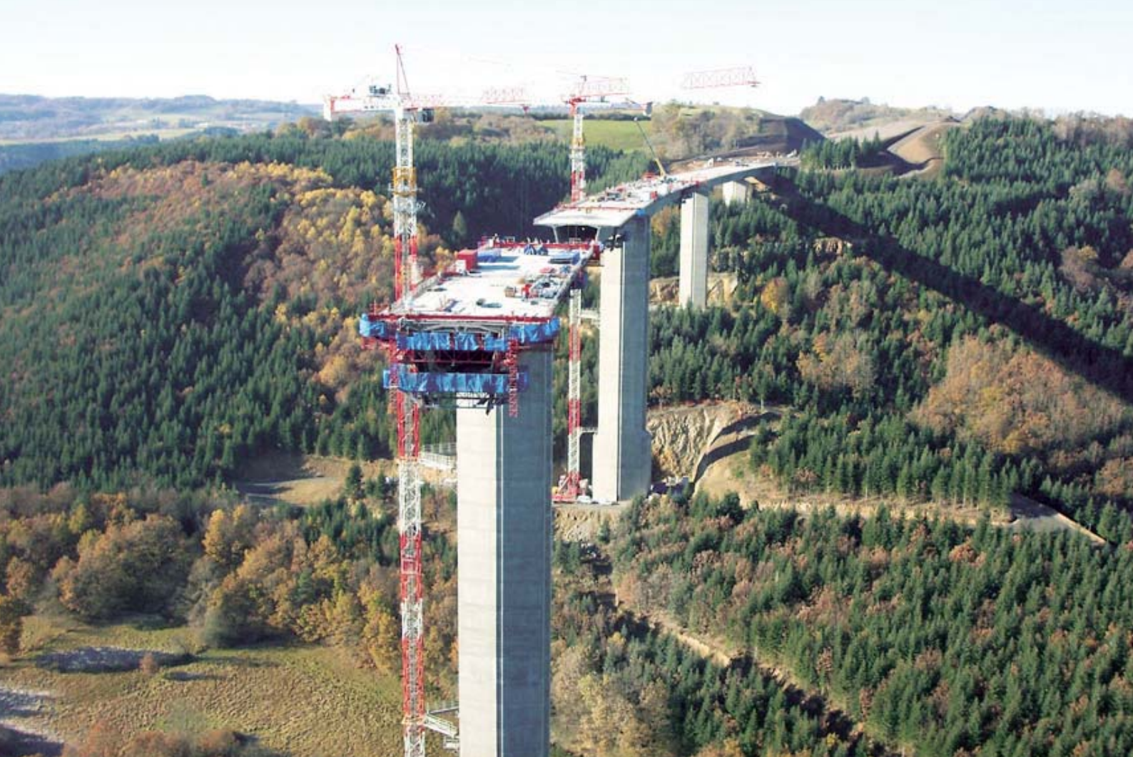
Sioule Viaduct on the A89.
