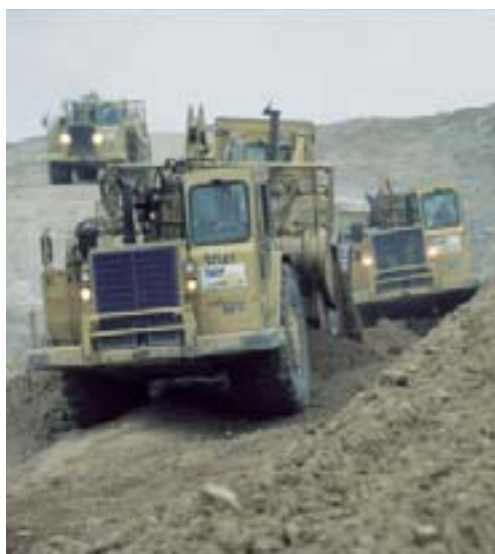
Construction of the A87.
