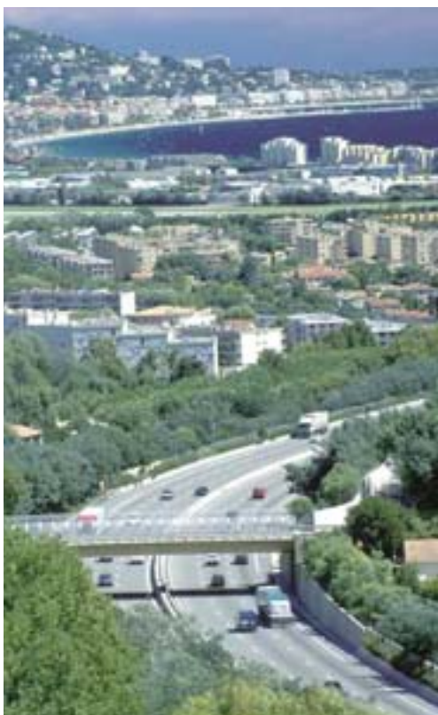
The A8 motorway (ESCOTA network).
