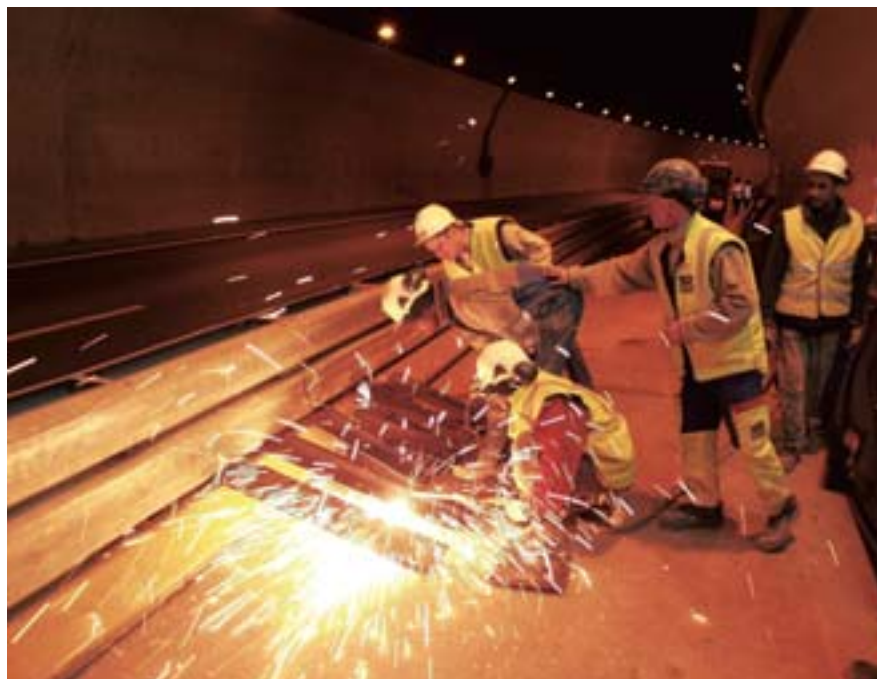
Work in a tunnel in the ESCOTA network.
