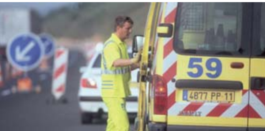
Working on the highway.
