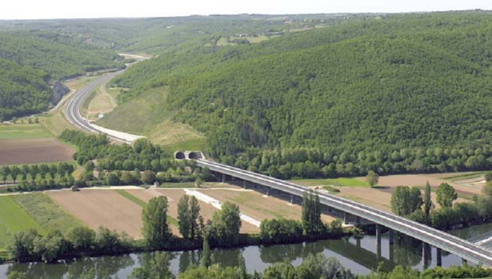
Lot Viaduct and La Garenne covered gallery on the A20.
